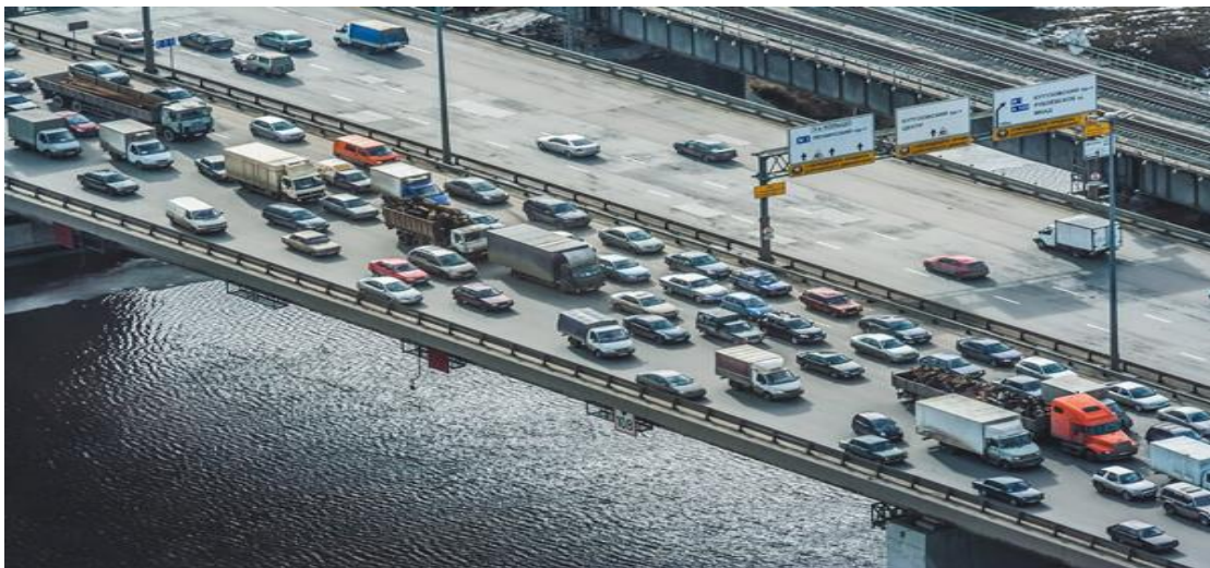
Figure 22 Example of a Traffic Bridge
