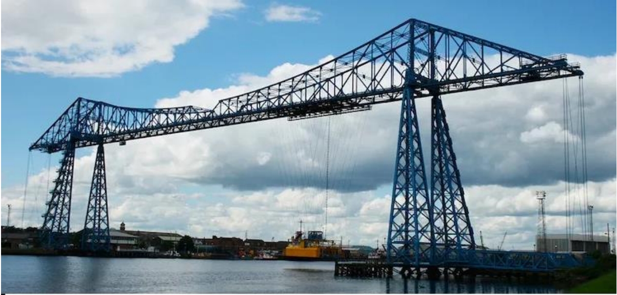
Figure 32 Middlesbrough Transporter Bridge Built in 1911
