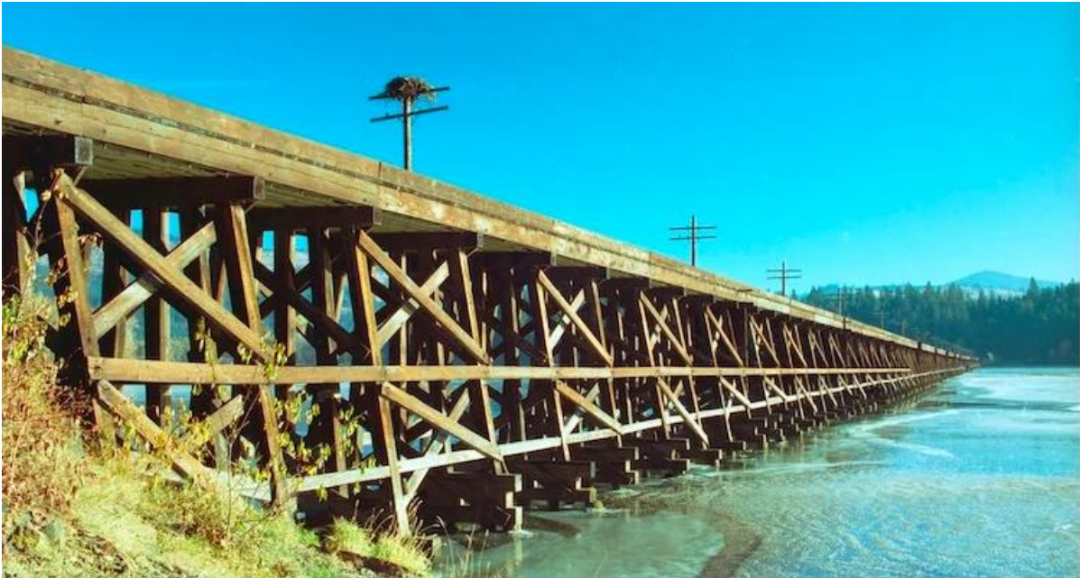
Figure 35 Montana Trestle Bridge
