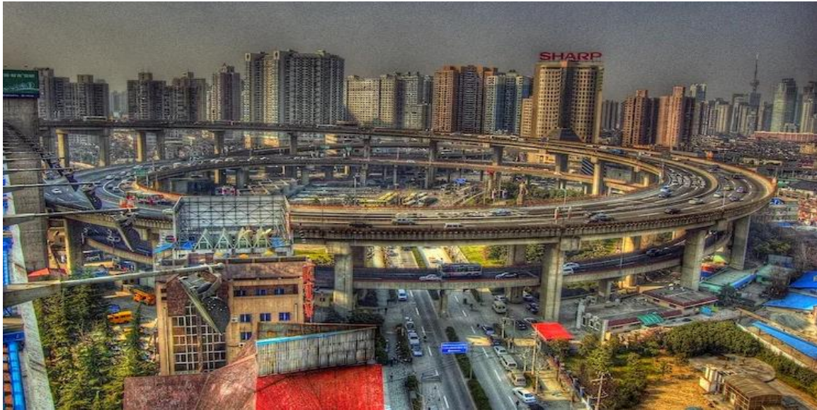
Figure 29 Spiral Ramp to Nanpu Bridge in Shanghai, China
