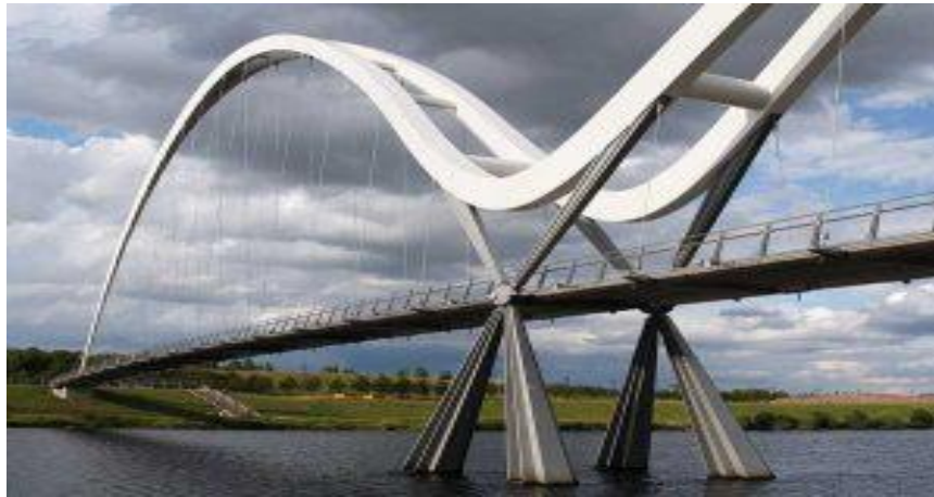
Figure 2 Example of a Tied Arch Bridge: Infinity Bridge in Stockton-on-Tees
