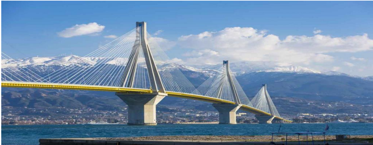
Figure 9 Example of a Cable-Stayed Bridge: The Rio Antirrio Bridge in Greece
