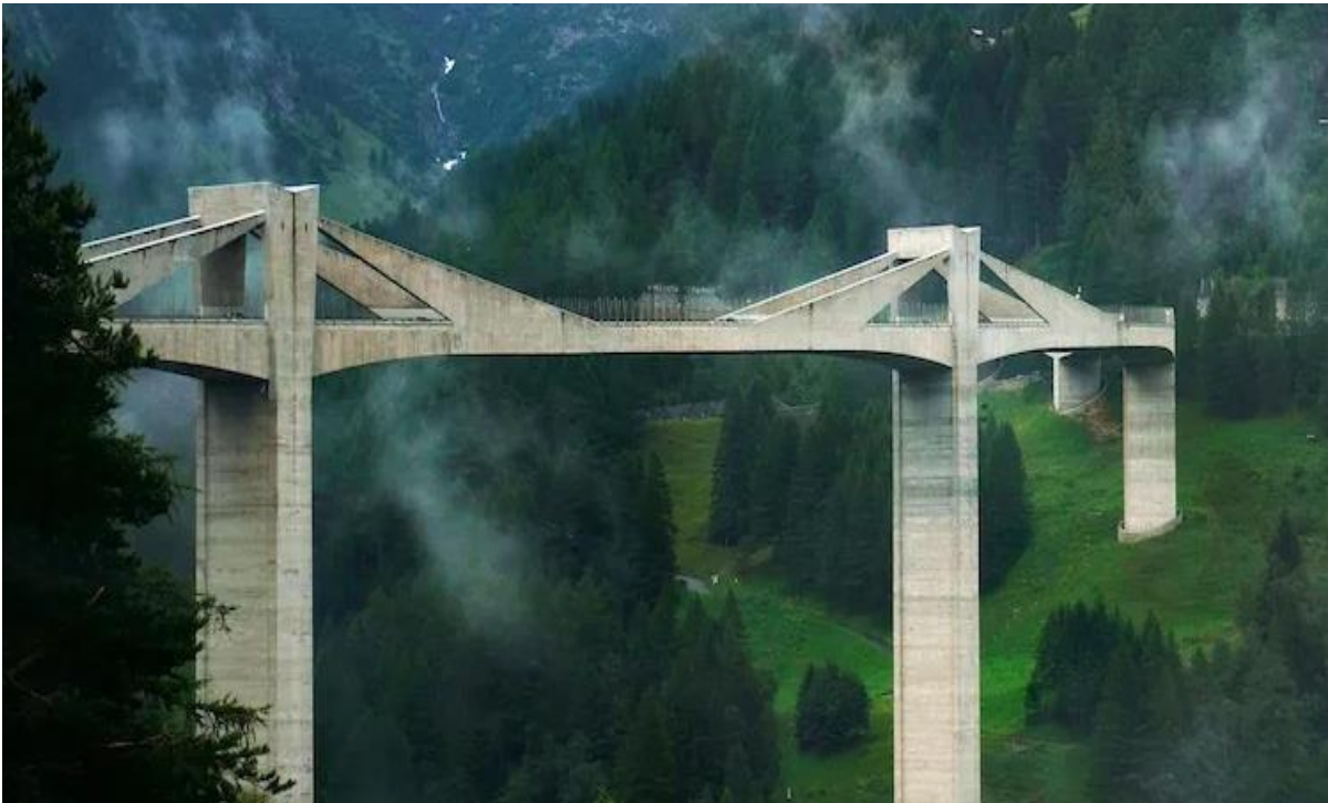
Figure 34 Ganter Bridge in Switzerland
