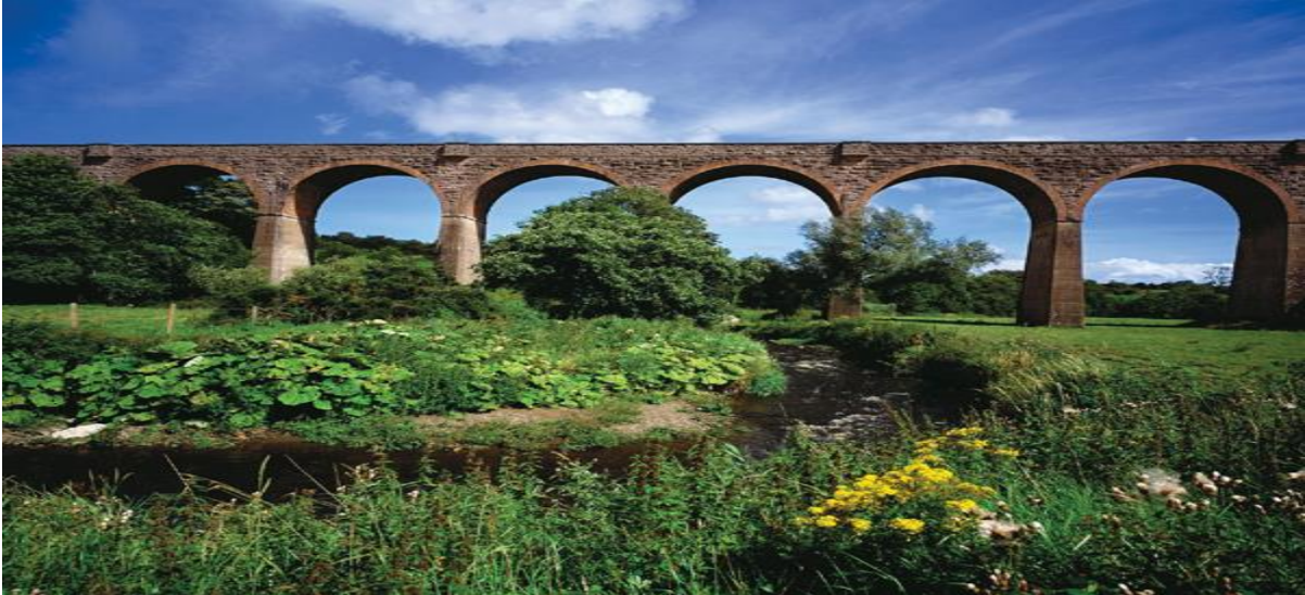
Figure 20 Example of an Aqueduct/Viaduct Pipeline Bridge
