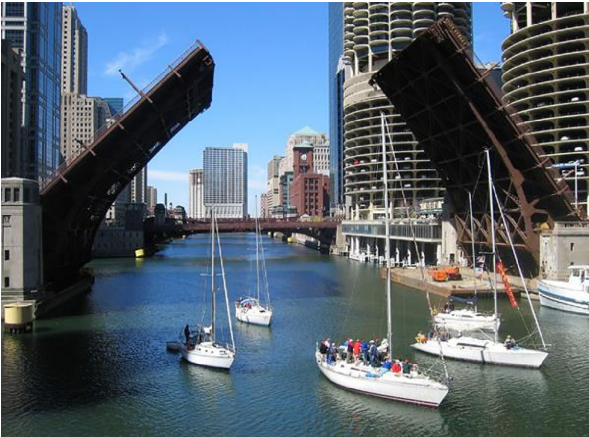
Figure 15 Example of a Movable Bridge
