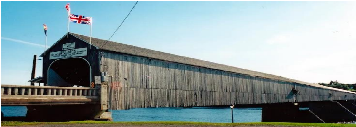
Figure 25 The Longest Covered Bridge is 1,282-feet Long | Hartland Bridge in New Brunswick
