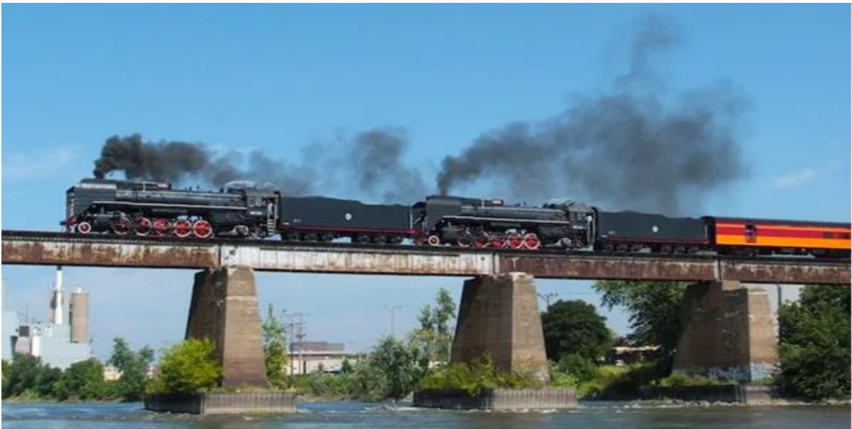
Figure 33 Multi-Span Plate Girder Bridge Deck on Concrete Piers
