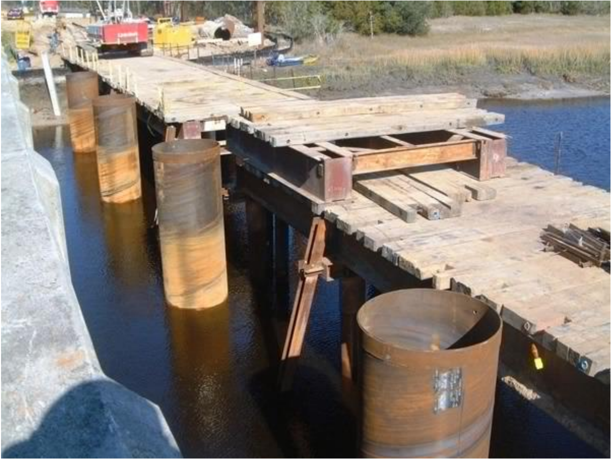
Figure 14 Example of a Temporary Bridge
